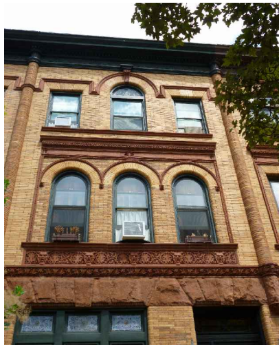
Top Half of Front Facade - Facing Decatur St
