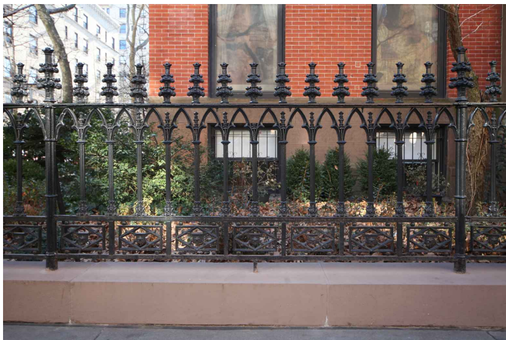
A Gothic Revival wrought iron fence
