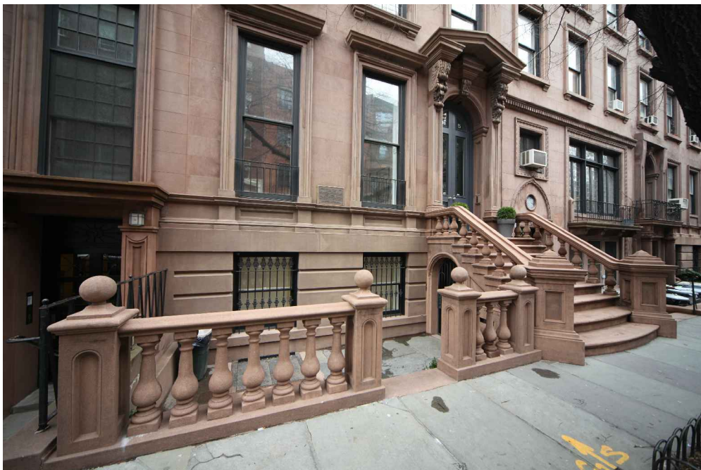
Brownstone stoop and areaway fence on an Italianate style rowhouse
