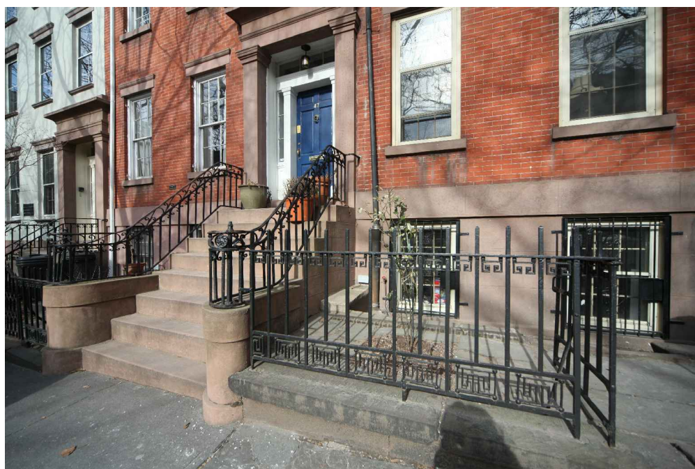
Wrought iron areaway fence and stoop rails on a Greek Revival style rowhouse
