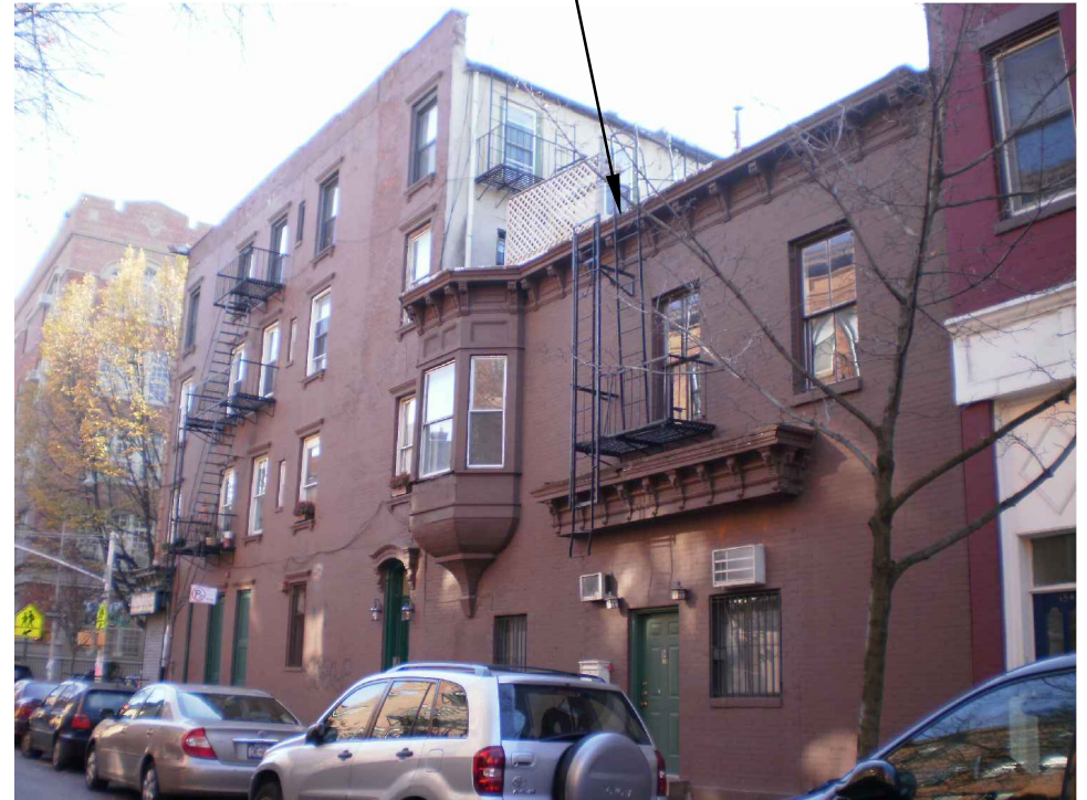
Taken from Crosby Street looking towards Howard Street and the rear elevation of the project site
