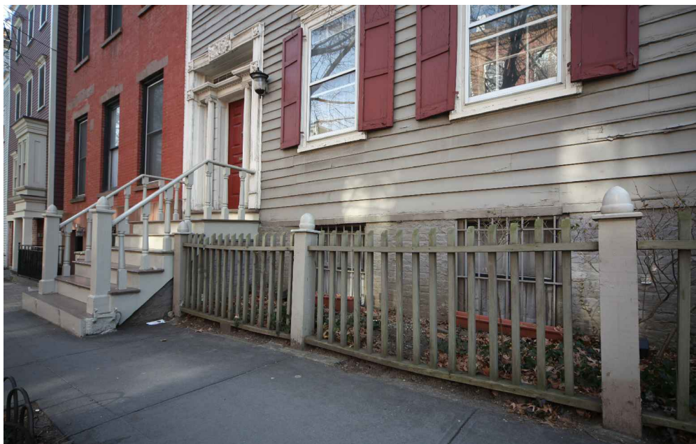
Wood fence, stoop and railings on a Federal style rowhouse
