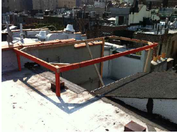
One example of a mock-up for a roof bulkhead
