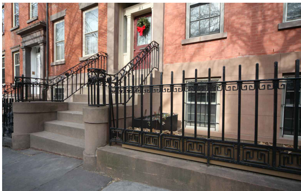
Wrought iron areaway fence and stoop rails on a Greek Revival style rowhouse
