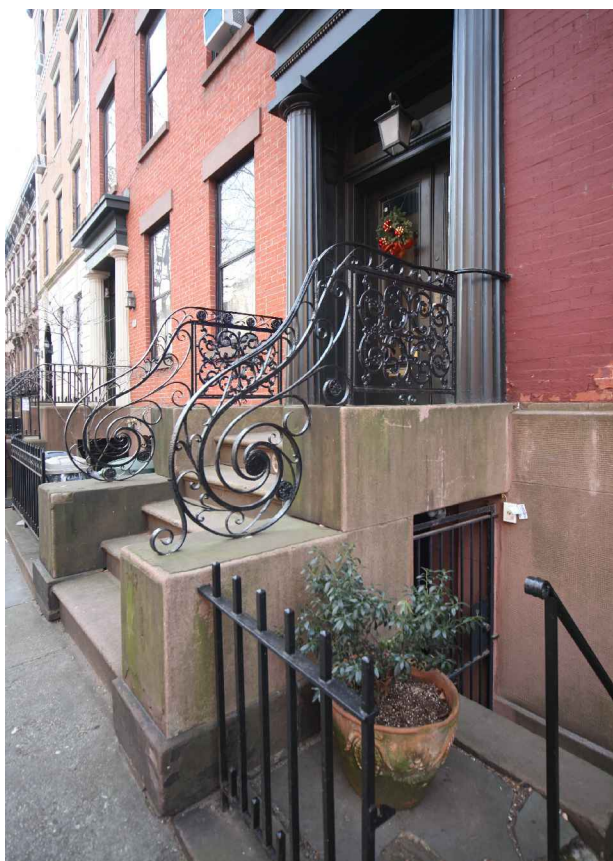
Wrought iron areaway fence and stoop rails on a Greek Revival style rowhouse
