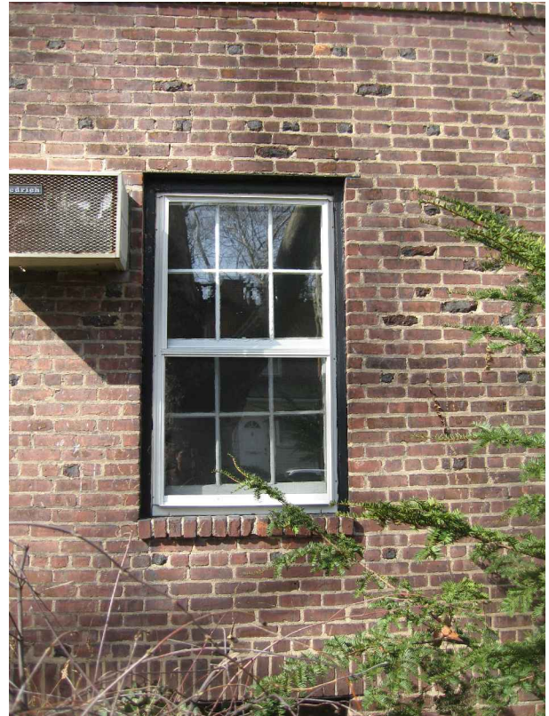
Exterior storm windows painted to match window sash
