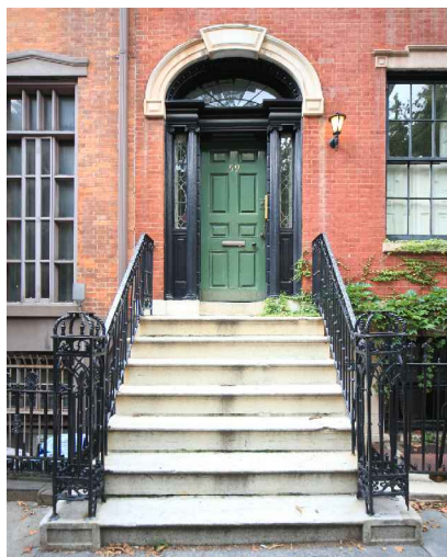
Example of an approved light fixture near an entryway
