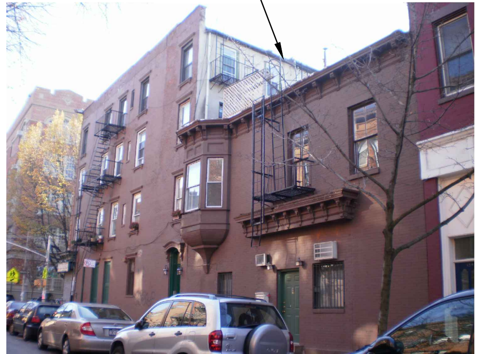
Taken from Roark Avenue looking towards Howard Street and the rear elevation of the project site
