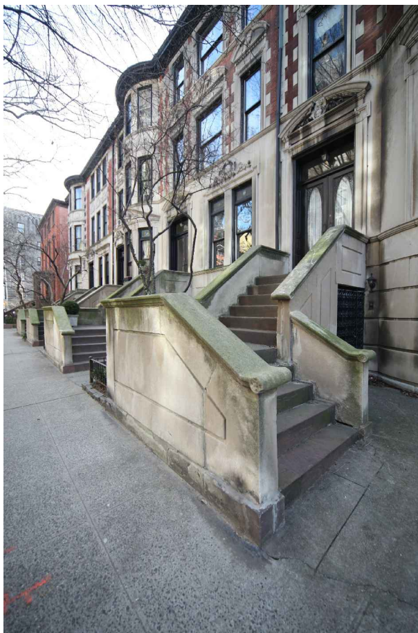
Limestone L-shaped stoop on a Renaissance Revival style rowhouse
