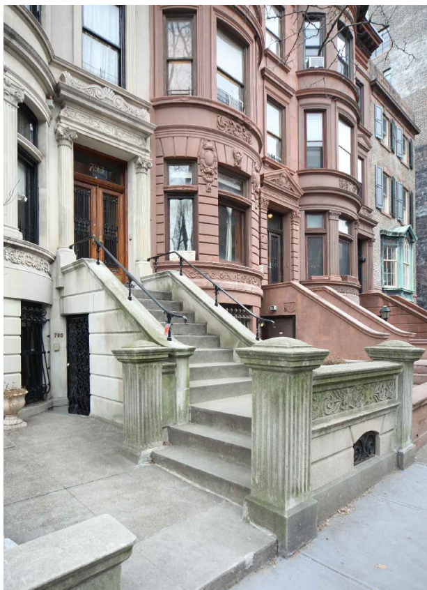
Limestone L-shaped stoop on a Renaissance Revival style rowhouse
