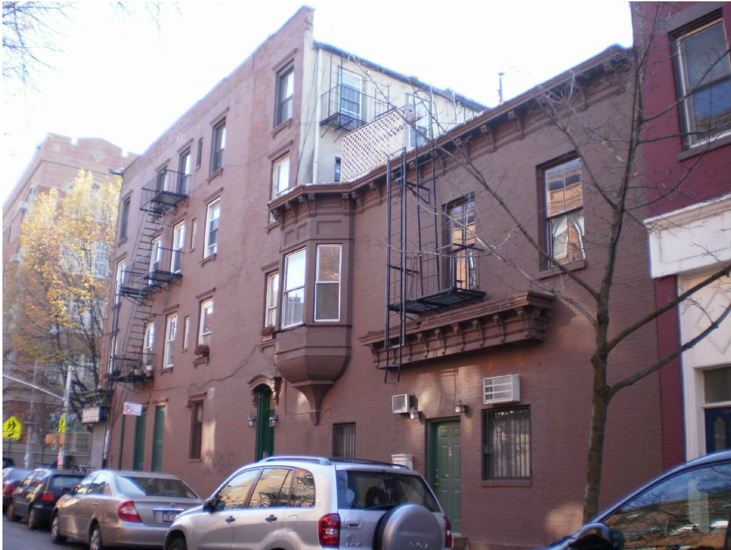
Adjacent Buildings on Crosby Street
