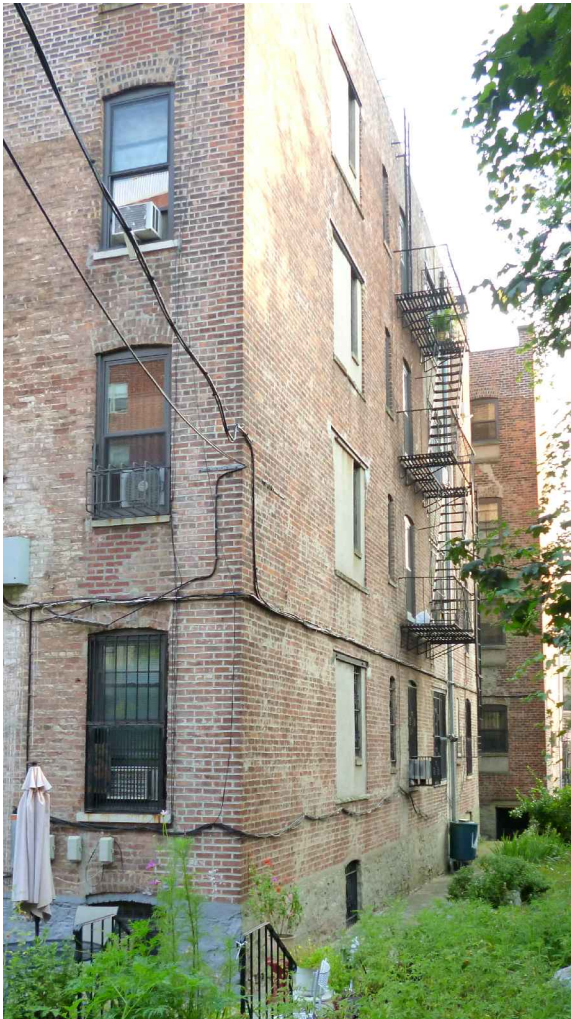
Replacement windows on a visible and non-visible secondary facade
