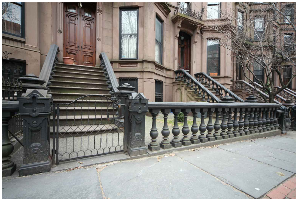
Cast iron areaway fence and stoop rails on a neo-Grec style rowhouse
