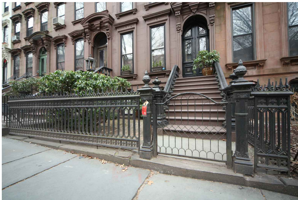
Cast iron fence and stoop rails on an Italianate style rowhouse
