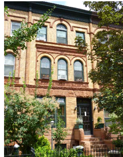
Front Elevation - Facing Decatur St
