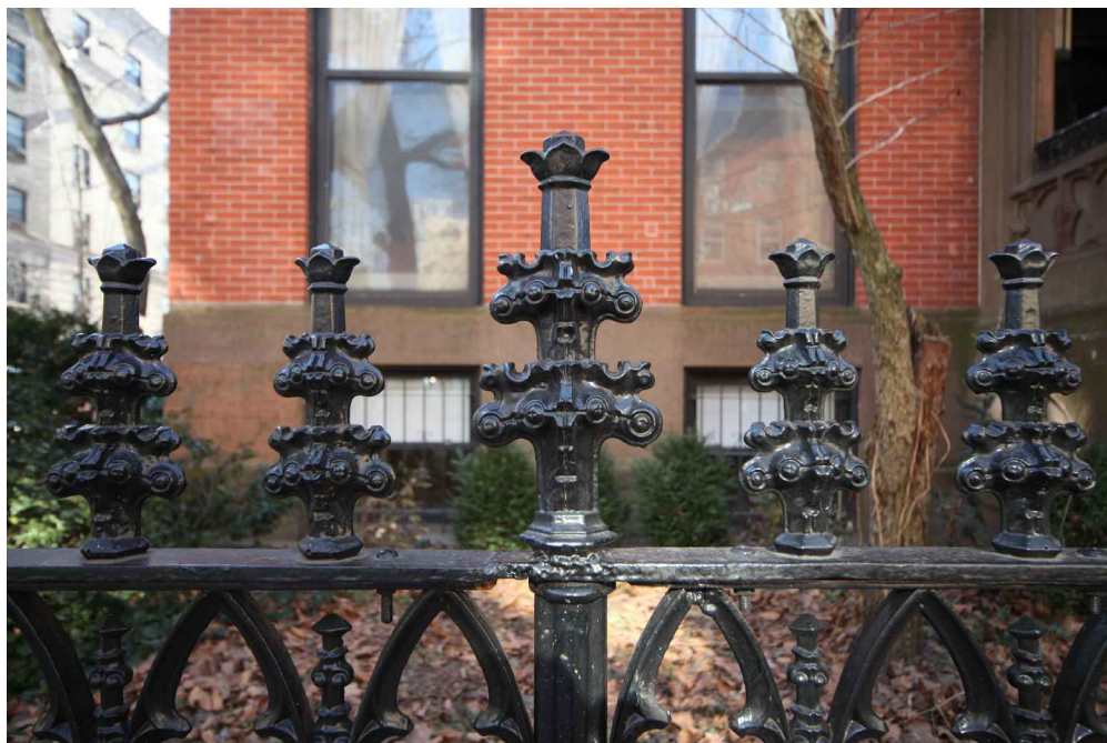
A Gothic Revival wrought iron fence
