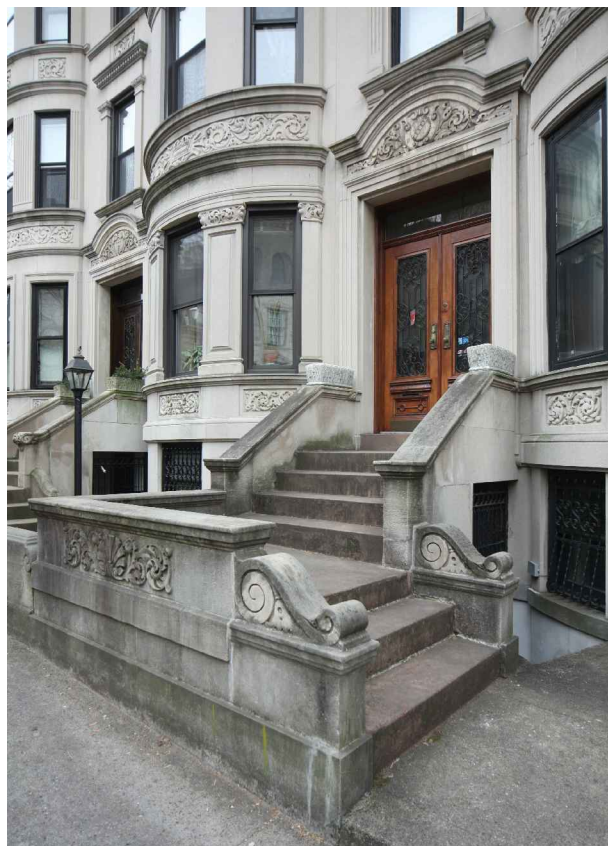
Limestone L-shaped stoop on a Renaissance Revival style rowhouse
