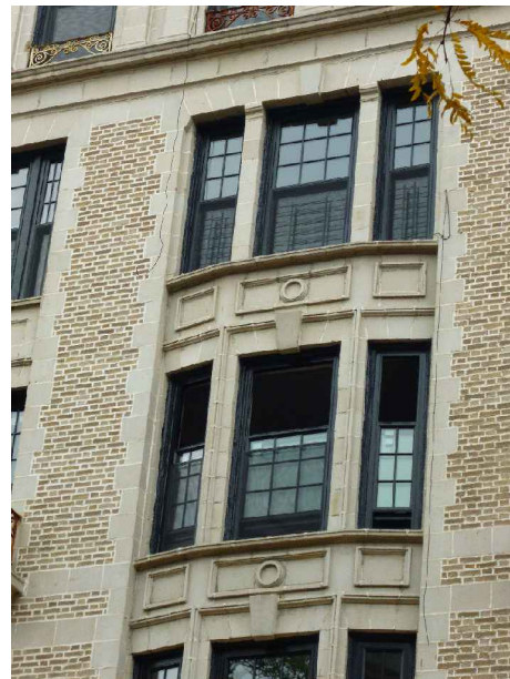
Replacing window sashes on the principal facade of a landmarked building with replacements of the correct historic configuration. (Photo at left, before. Photo at right, after)
