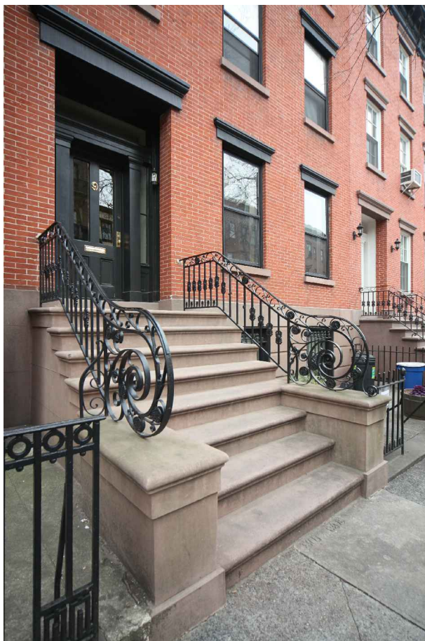
Wrought iron areaway fence and stoop rails on a Greek Revival style rowhouse
