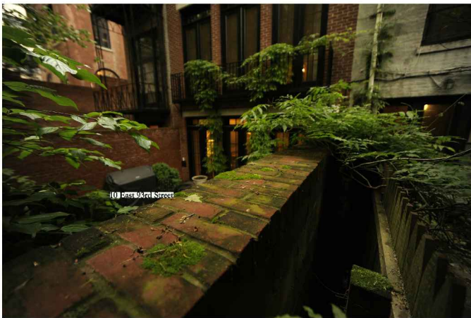
PHOTO 8 - REAR FACADE 10 East 93rd Street
